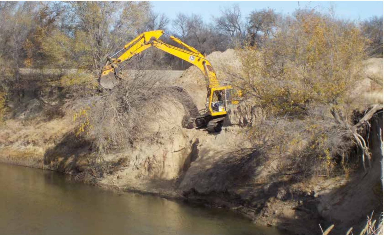
BACKHOE ON STREAMBANK INSTALLING TREES
