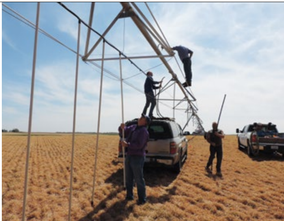
INSTALLING TEST STRIPS AT WATER TECHNOLOGY FARM — THREE OUTER SPANS HAVE HALF-MOBILE DRIP IRRIGATION AND HALF MID-ELEVATION SPRAY APPLICATION.
